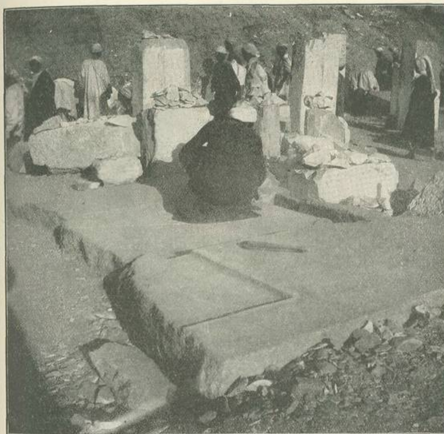
THE GRANITE THRESHOLD AND OCTAGONAL SANDSTONE PILLARS OF THE Xth DYNASTY TEMPLE AT DÊR EL - BAHARI.
